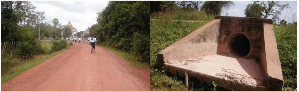
The paths and water piper build in 2012 at Roeul commune by commune development budget, Siem Reap province.
